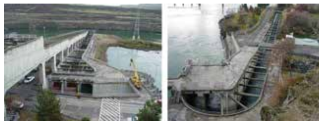
Figure 4. The Dalles Dam on the Columbia River has both an east ladder (left) and north ladder (right). The wider east ladder passed more sturgeons. Photo credits: U.S. Geological Survey.
