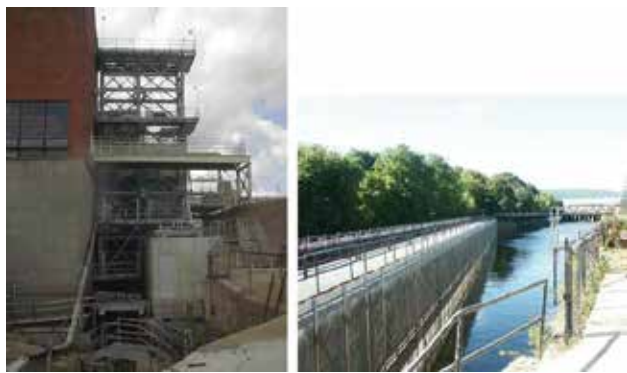
Figure 3. Fish passage facilities at Hadley Falls at the Holyoke Project on the Connecticut River. A fish lift is used to transport anadromous sturgeons upstream (left), and a large bypass canal permits return downstream (right). Photo credit: Duchenev et al. (2006).
